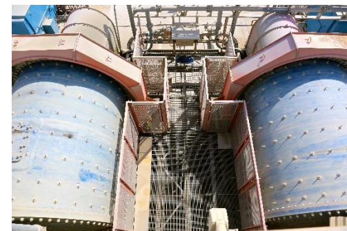
NLGM Processing Plant
