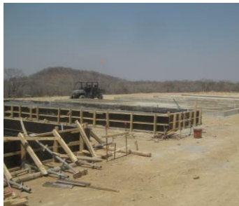
Power station foundations
