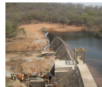
Luika River dam
