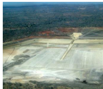
Tailings Storage Facility
