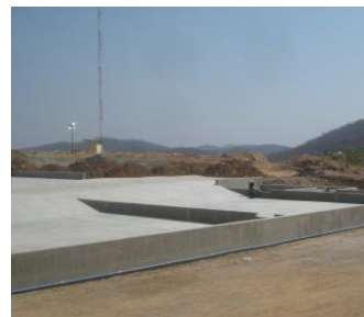
Underground Settling Pond
